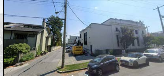
2. ADDITION TO HISTORIC BANK FROM LANE
