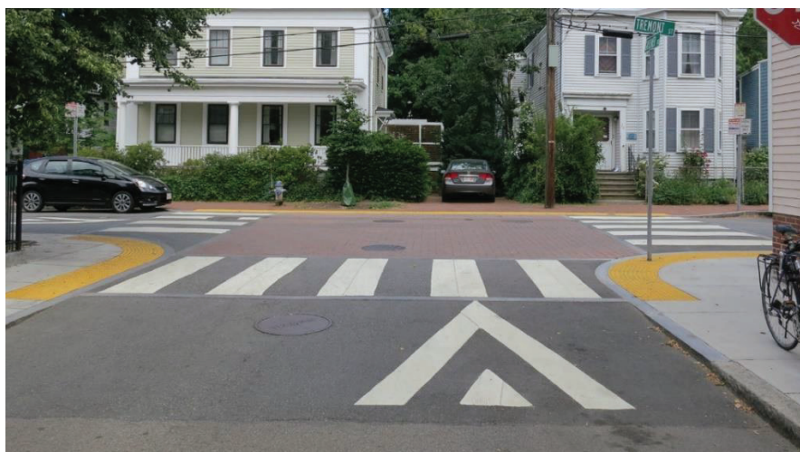
Figure 26. Example of Raised Intersection Treatment
