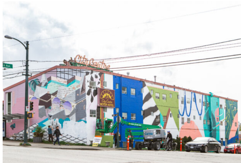
Looking south from E 5th Ave
