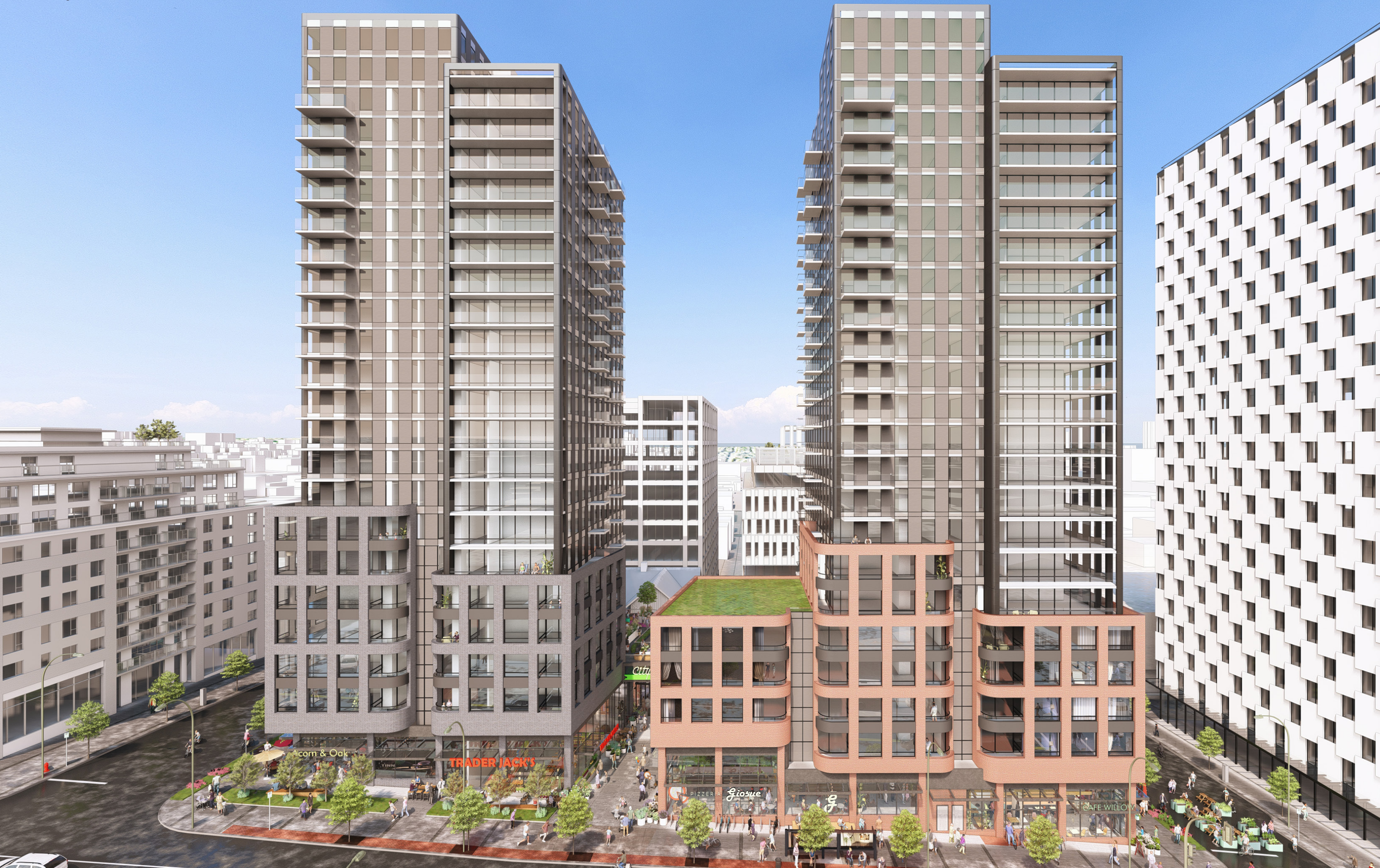
View looking southwest to site
