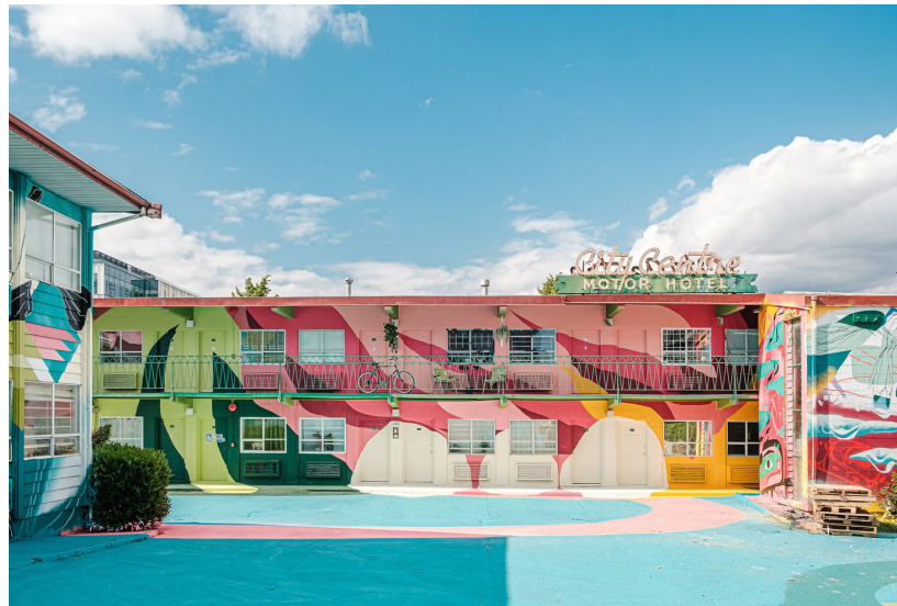
View looking north from E 6th Ave
