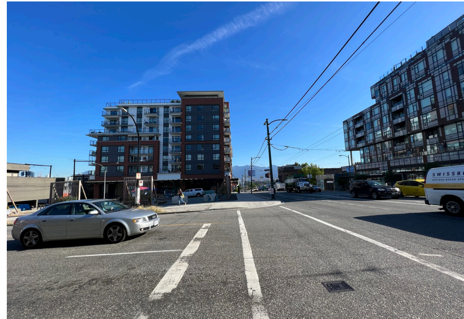
View looking north from E 7th Ave.
