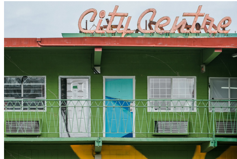
Looking north from interior courtyard
