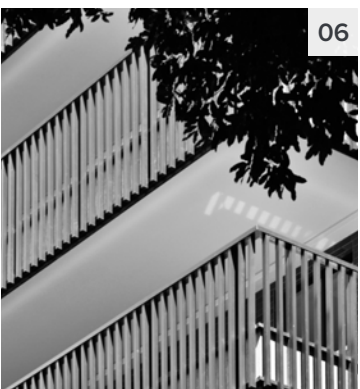
Vertical face mounted picket style guardrails at podium
