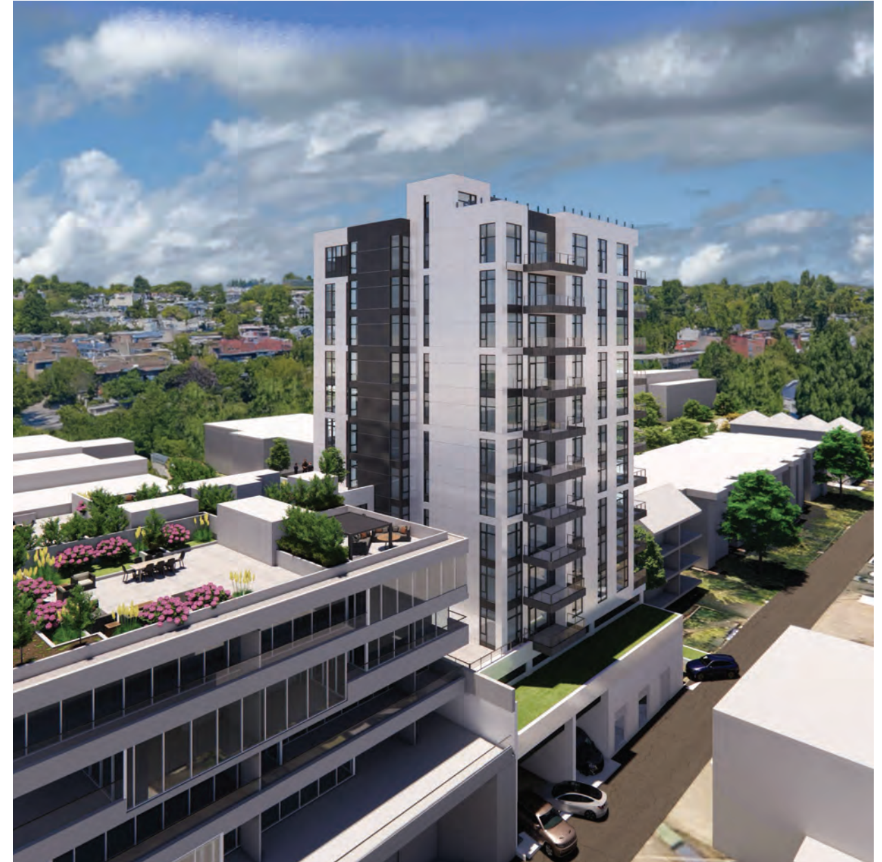
Aerial view from lane towards SW
