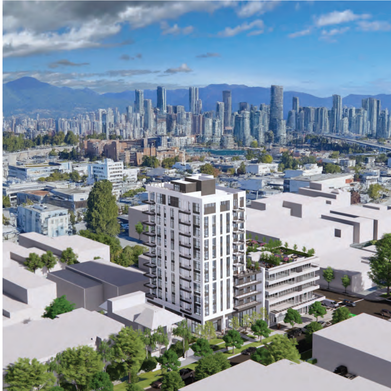
Aerial view towards NE
