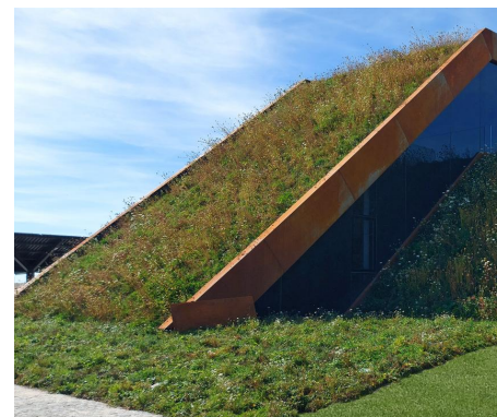
Sloped Green Roof
