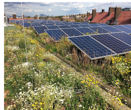
Upper Green Roof with PV Panels
