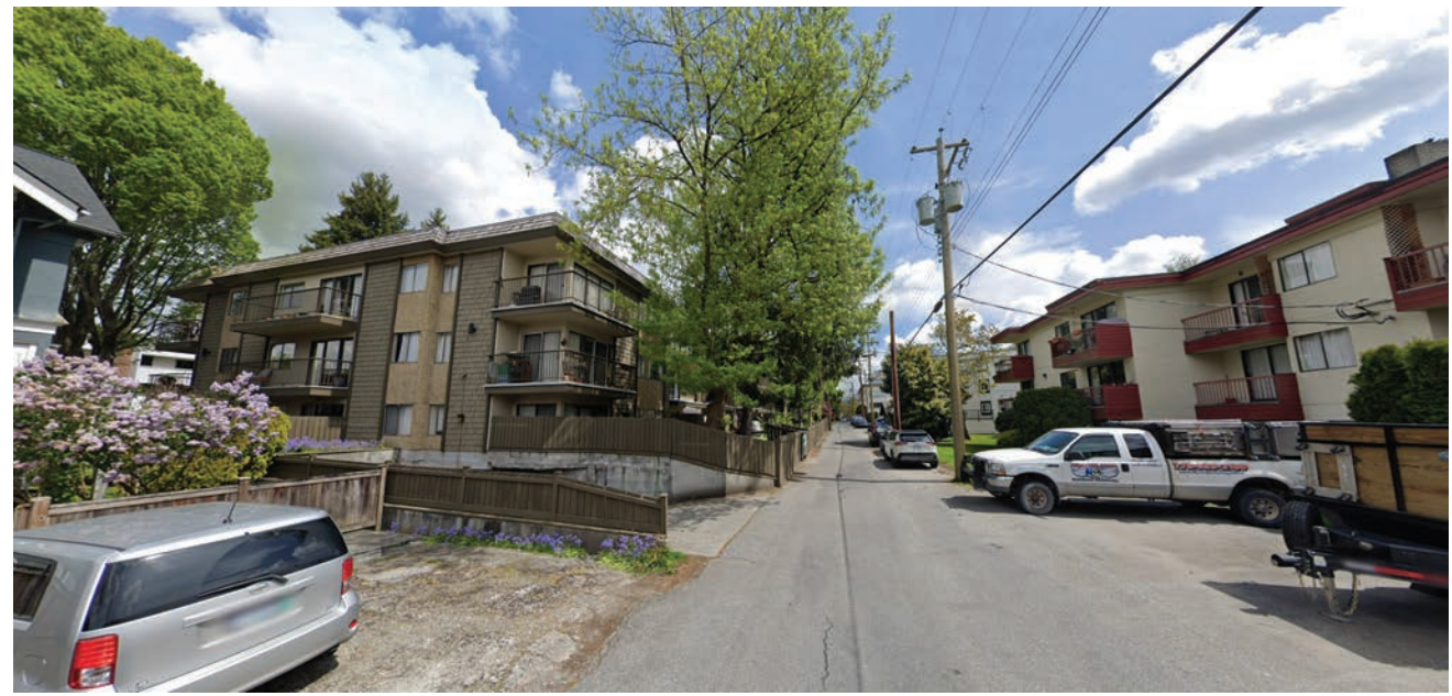
4. VIEW OF LANEWAY FROM SOUTH-WEST CORNER OF SITE
