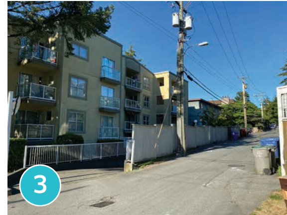
3 South view on Lane.
