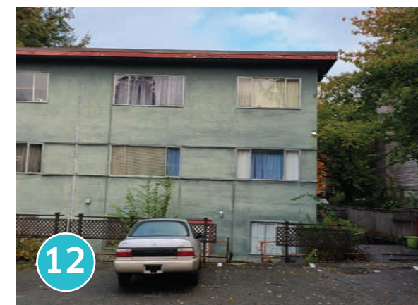
12 South view on Lane.
