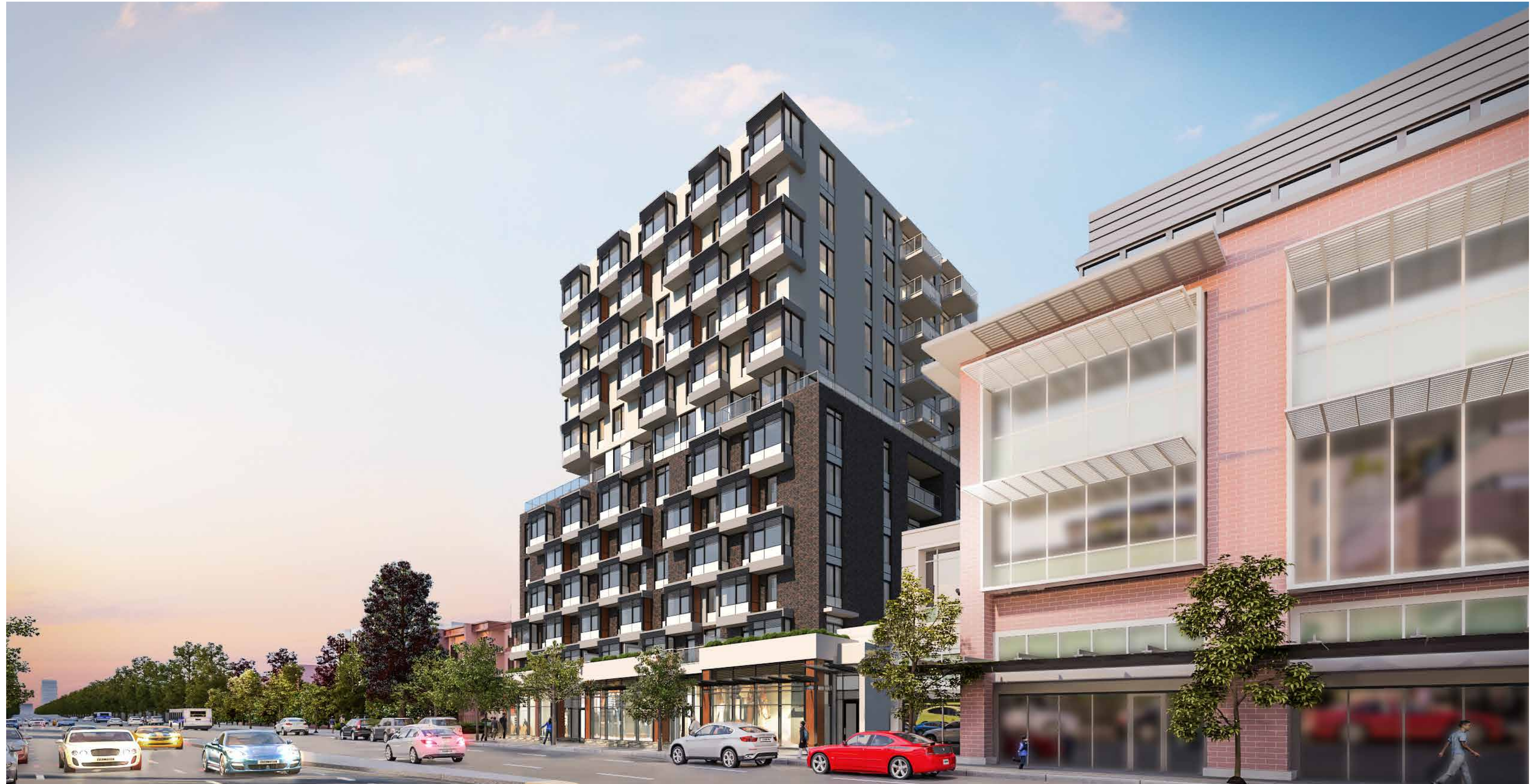
STREET VIEW FROM EAST BROADWAY LOOKING WEST
