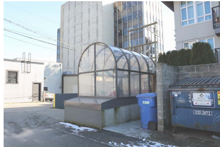
Parking and stair access from rear lane to 1551 West 11th Avenue
