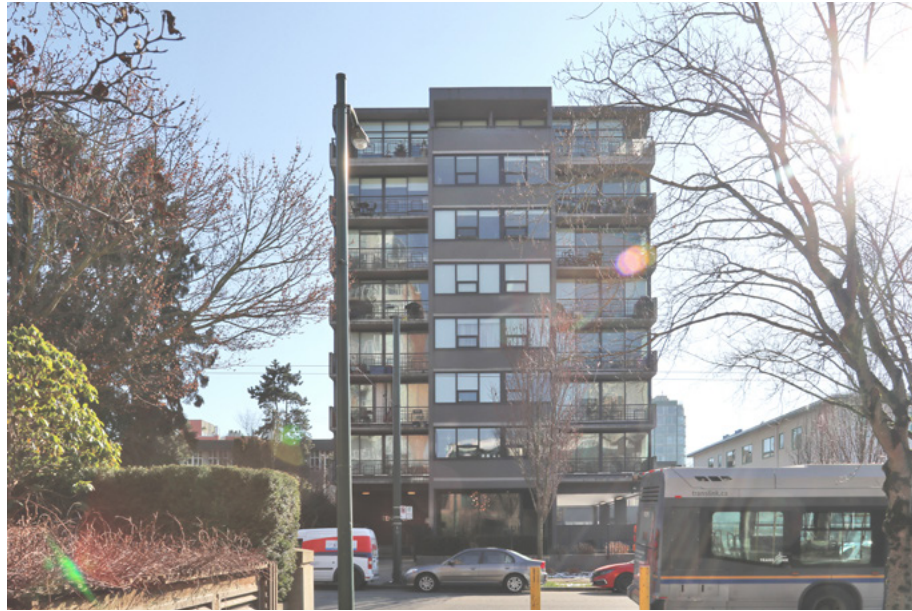
Neighbouring building (west), 1550 West 10th Avenue
