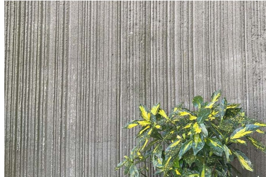
Brushed concrete at passageway
