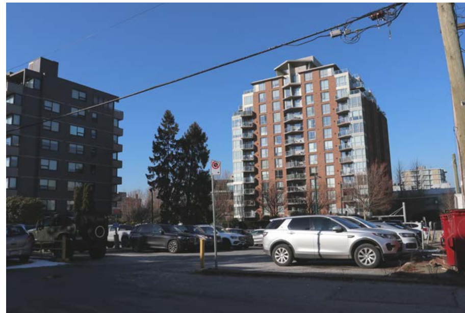
04 – View of site form southwest corner
