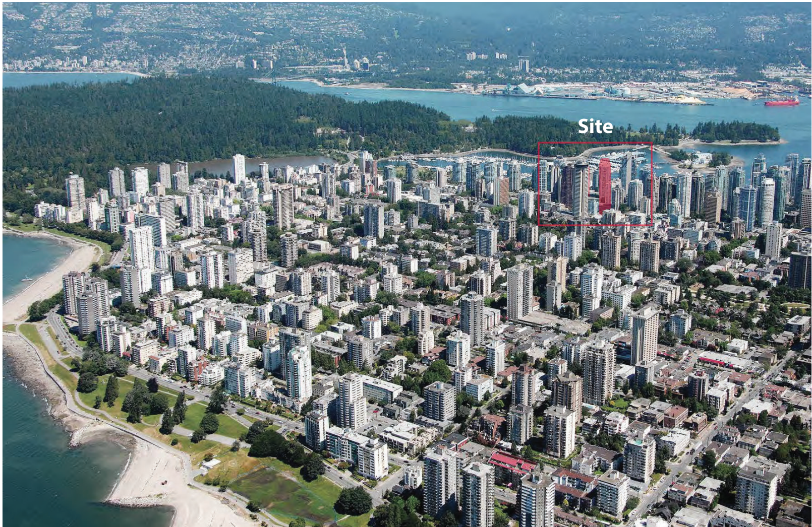
AERIAL VIEW OF WEST END
