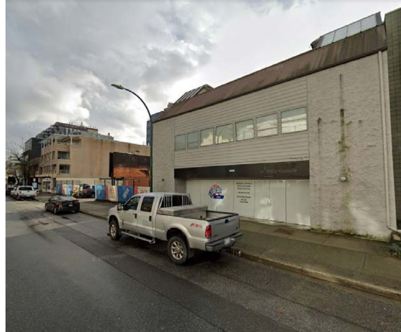
1. View looking southeast to the site from 8th Ave
