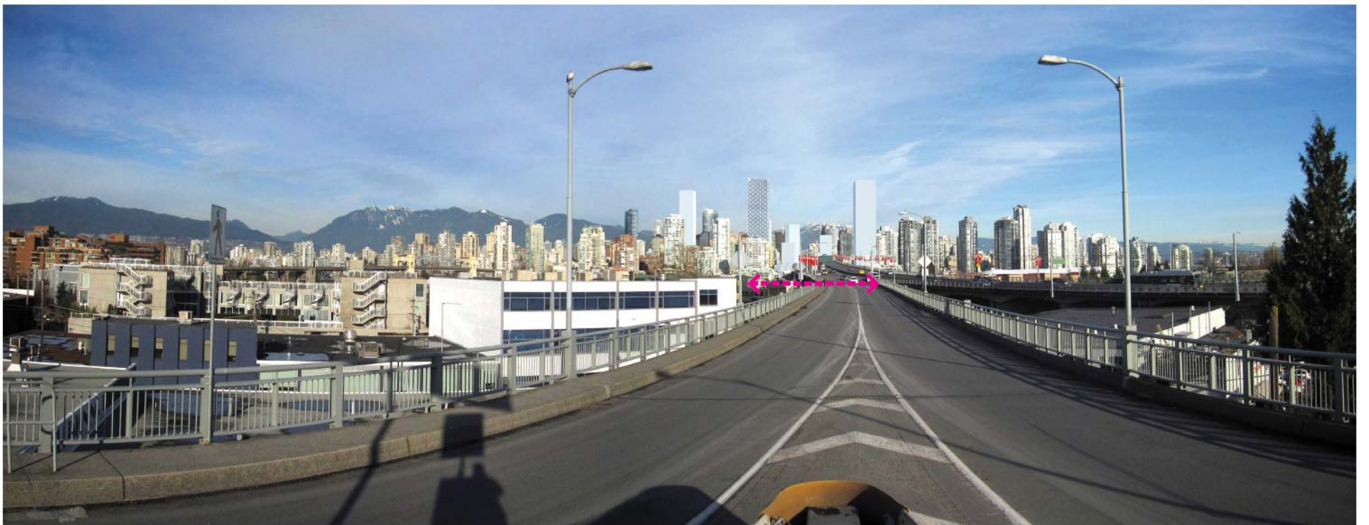
WEST-EAST SKYLINE COLLAGE. VIEW FROM SOUTH SIDE OF GRANVILLE BRIDGE BETWEEN W 3RD AVE/W 4TH AVE AND FIR ST/GRANVILLE ST
