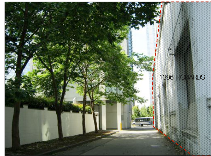
05. LANE LOOKING SOUTH
