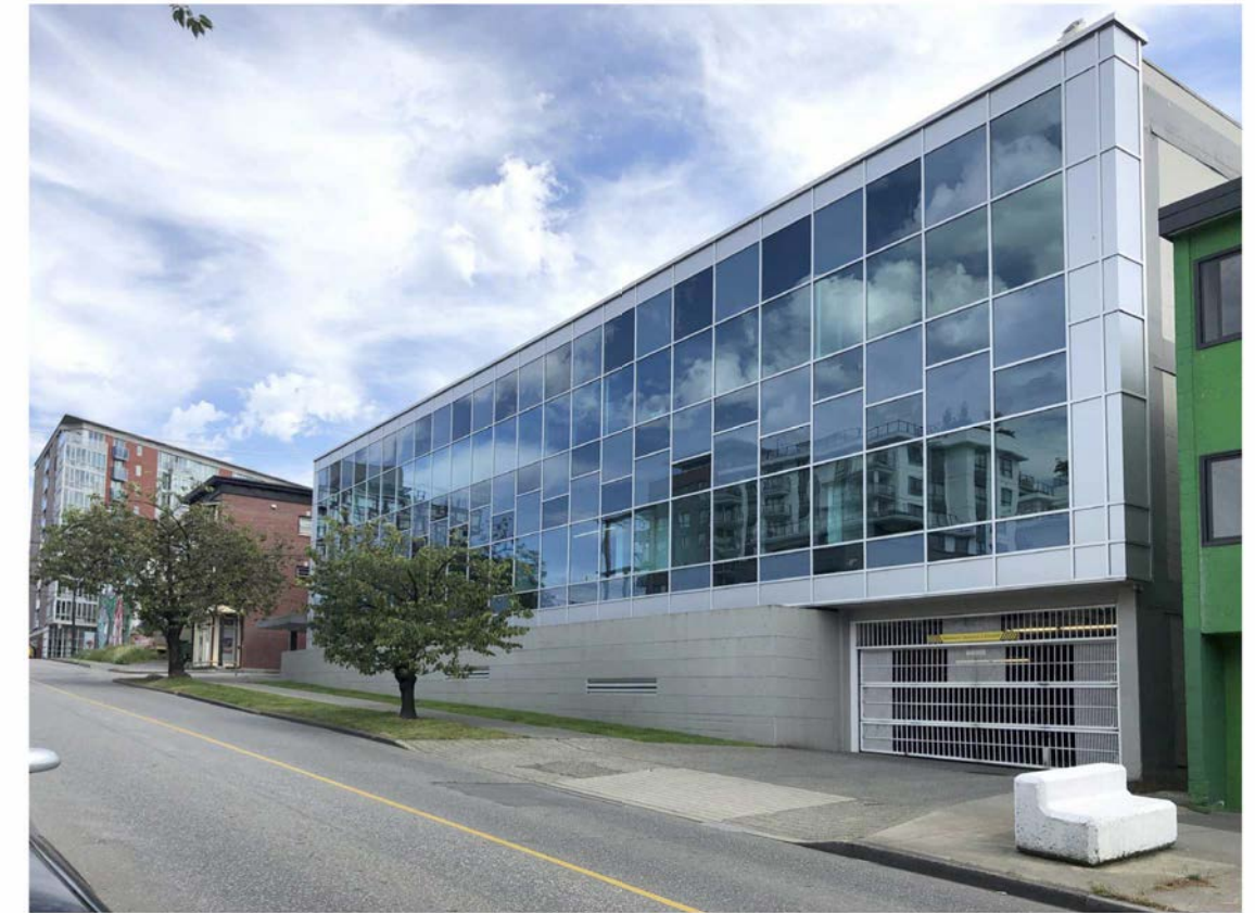
View looking from the North West corner
