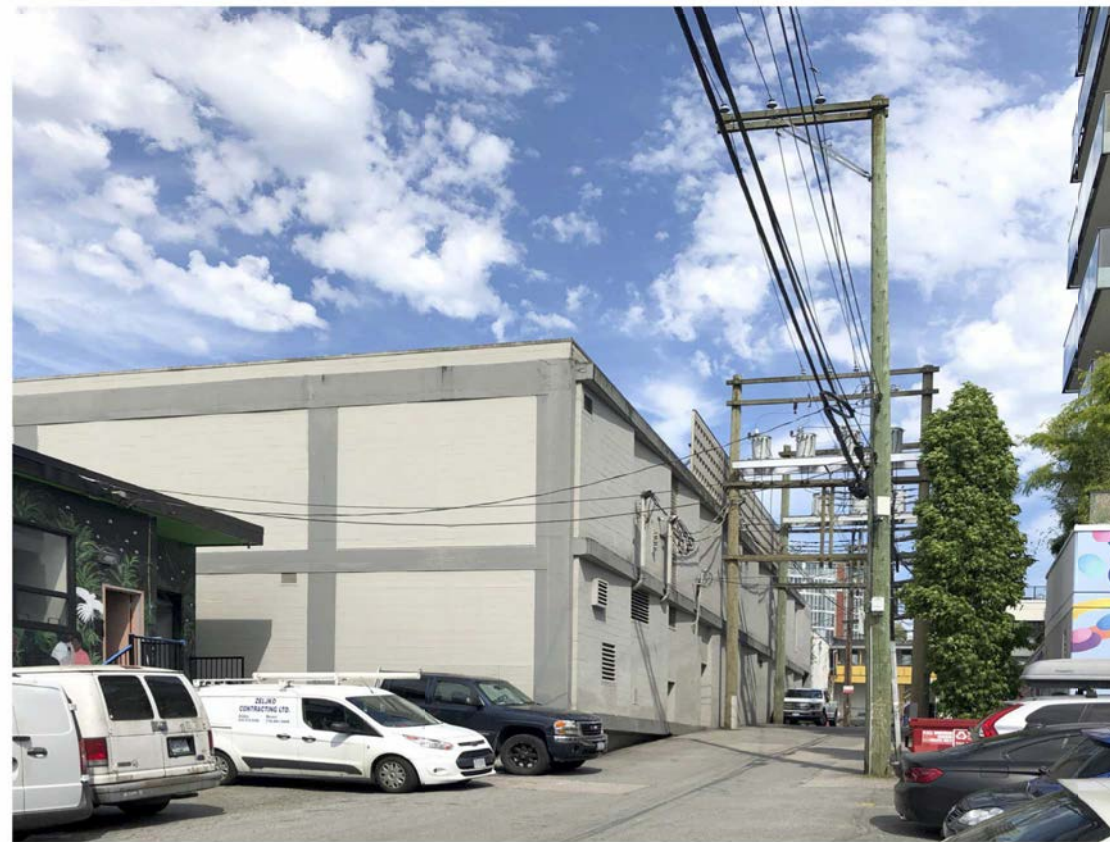
View looking from the South East corner
