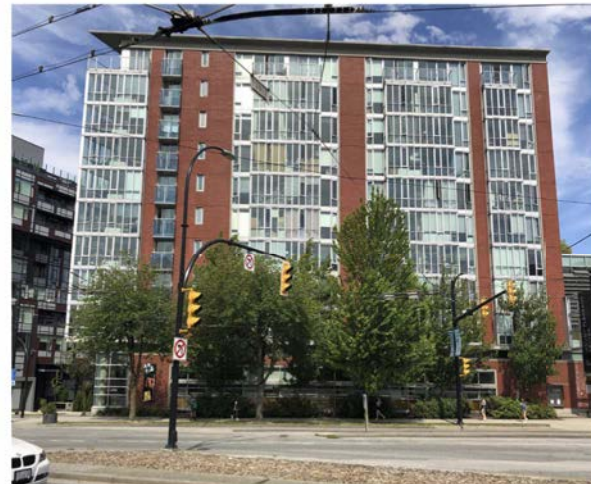
1 Kingsway Mount Pleasant Community Centre Vancouver Public Library - Mount Pleasant Branch (10 Storey - Cultural and Residential)
