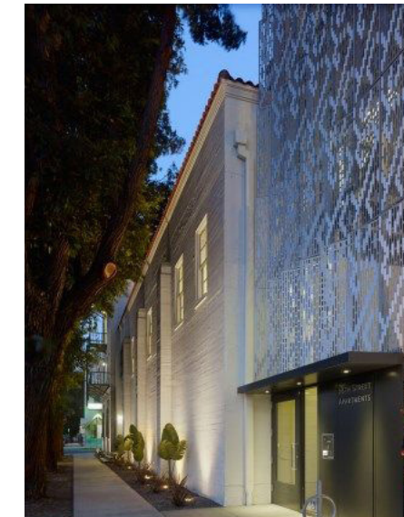
Feature lighting accents on facade
