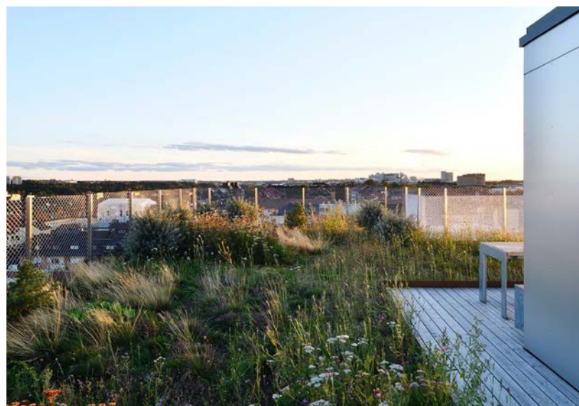
Extensive green roof planting
