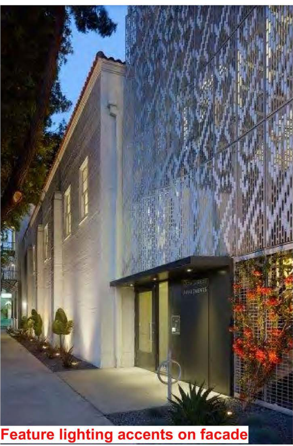
Feature lighting accents on facade
