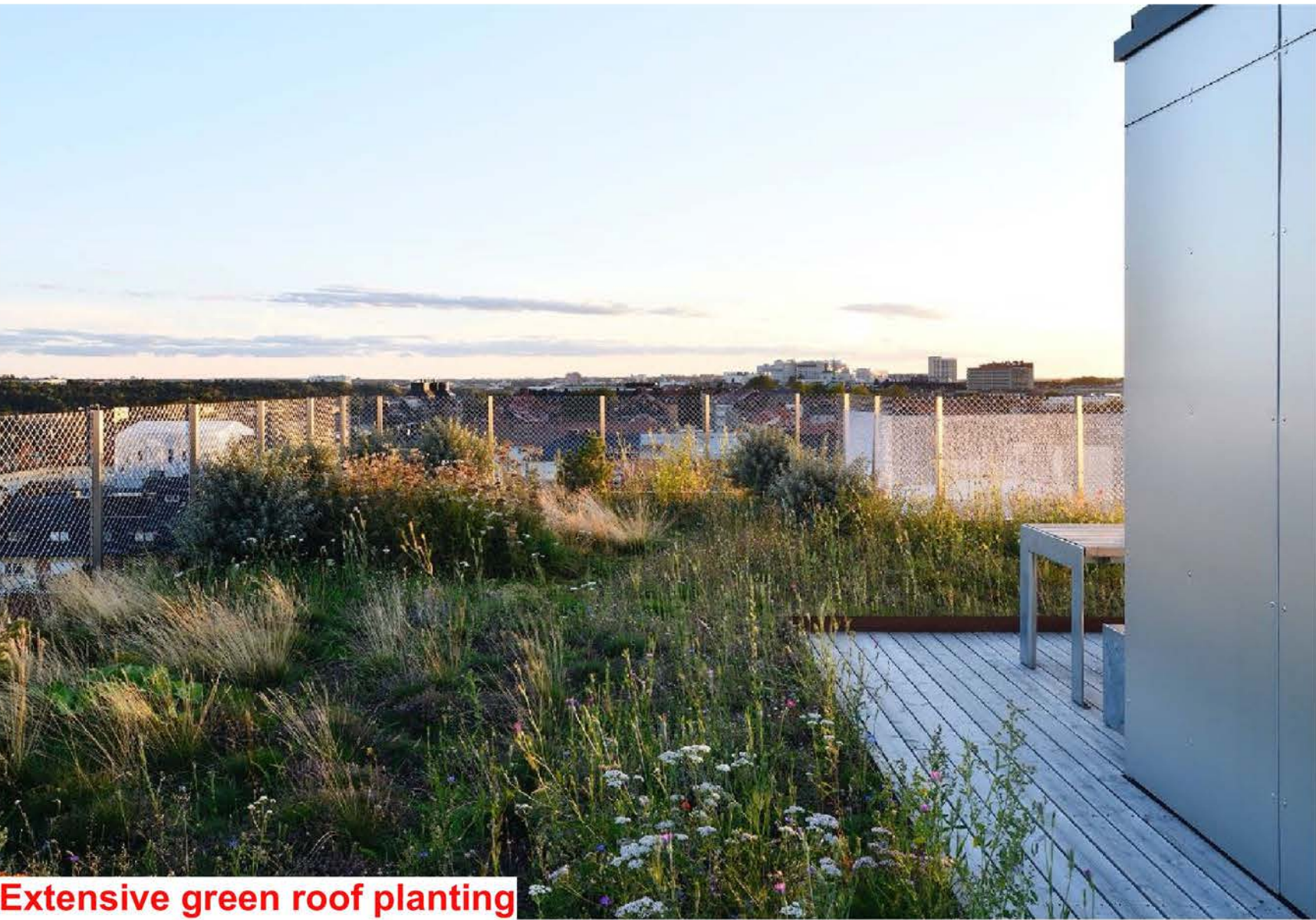
Extensive green roof planting
