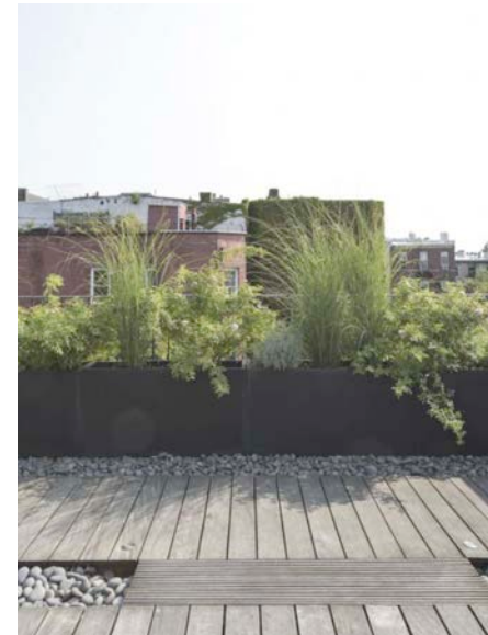
Planters at roof edge
