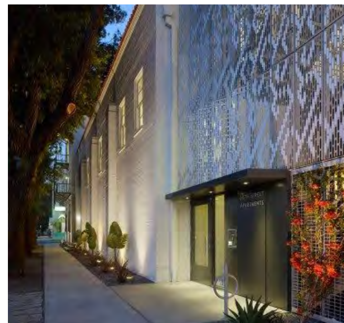
Feature Lighting Accents on Facade
