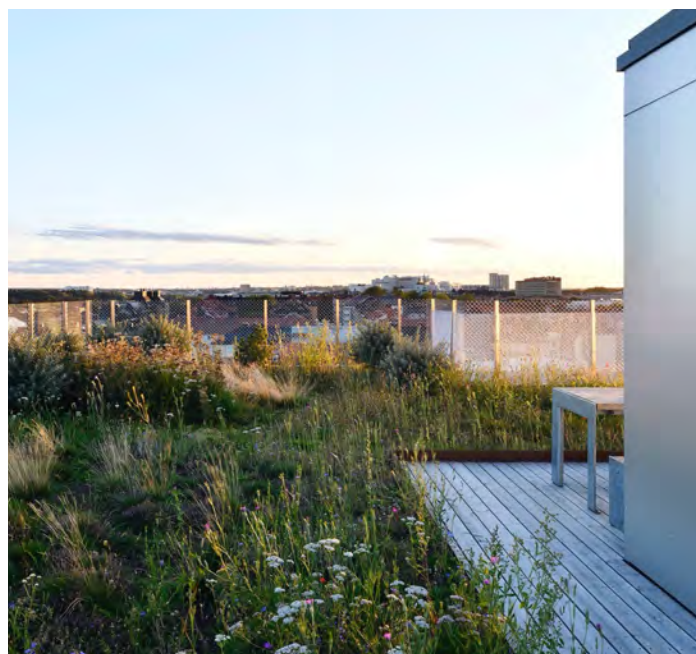
Extensive Green Roof Planting
