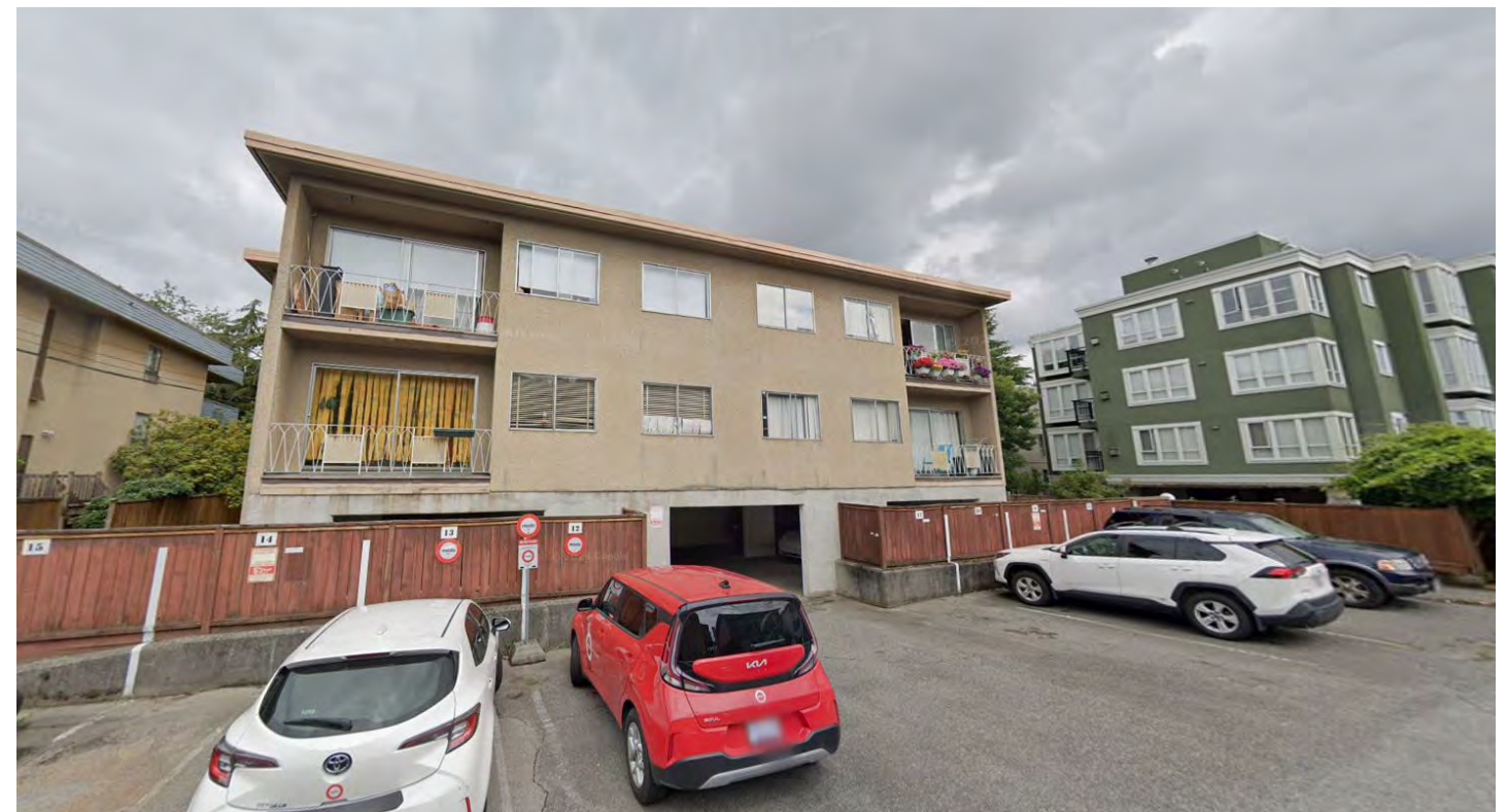
4. North View from South Lane
