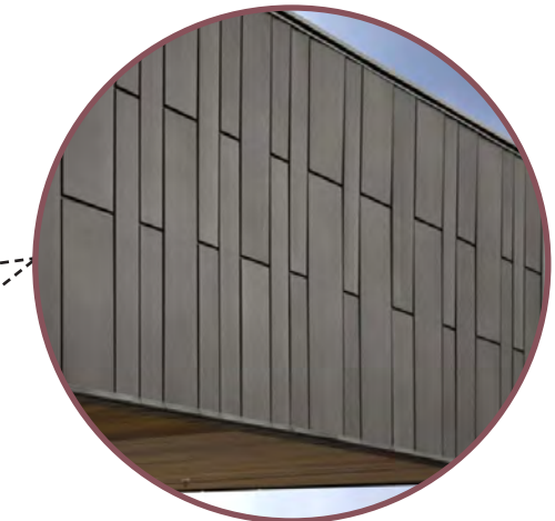
Metal / Cementitious Cladding
