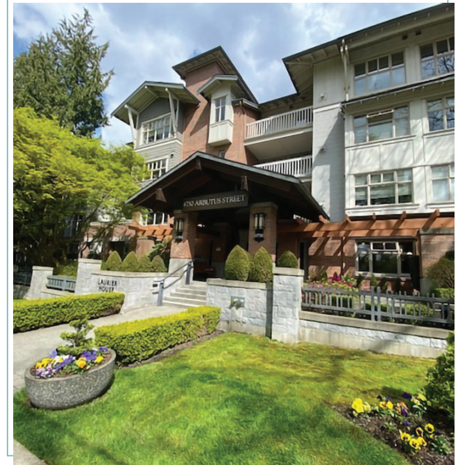
Project - Laurier House
