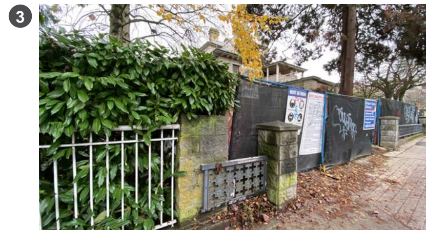
Existing interface at southeast corner with existing fence
