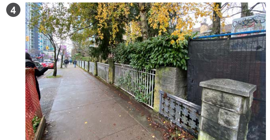
Significant grade drop from sidewalk to existing roots of tree to be maintained
