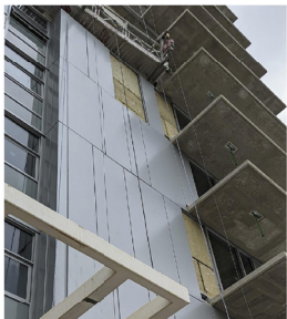
[3] window wall by TORO - raised metal panel - color match TE 10 powder coat
