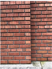
[4] existing brick facade
