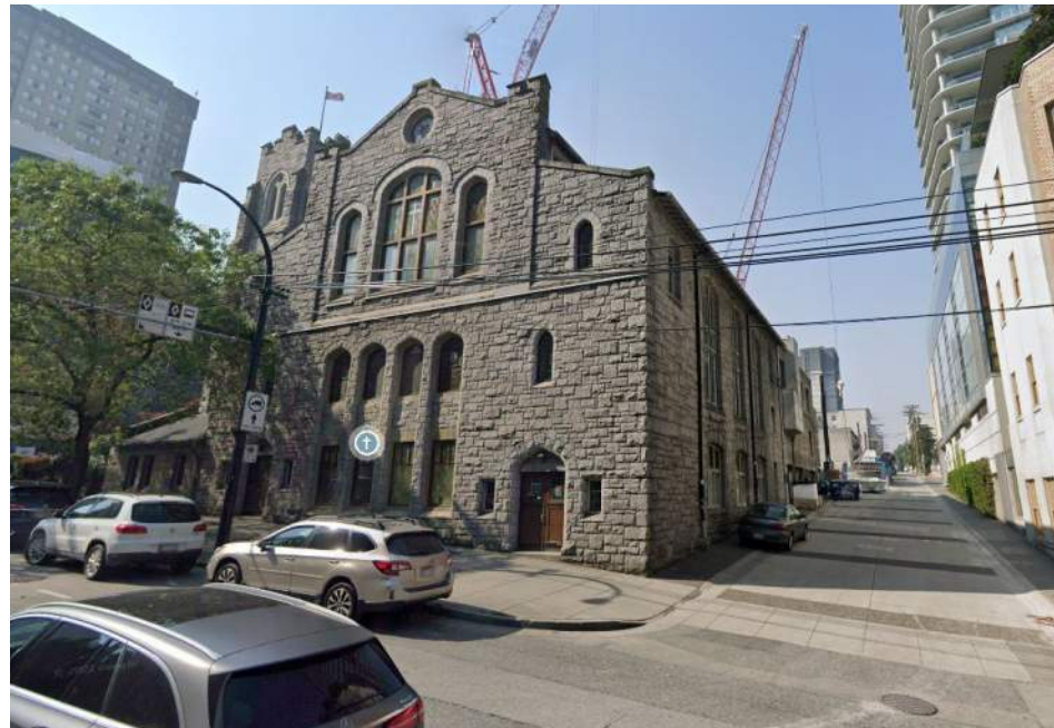
E. Burrard St and Ted Northe Ln frontages of the First Baptist Church at 969 Burrard St.
