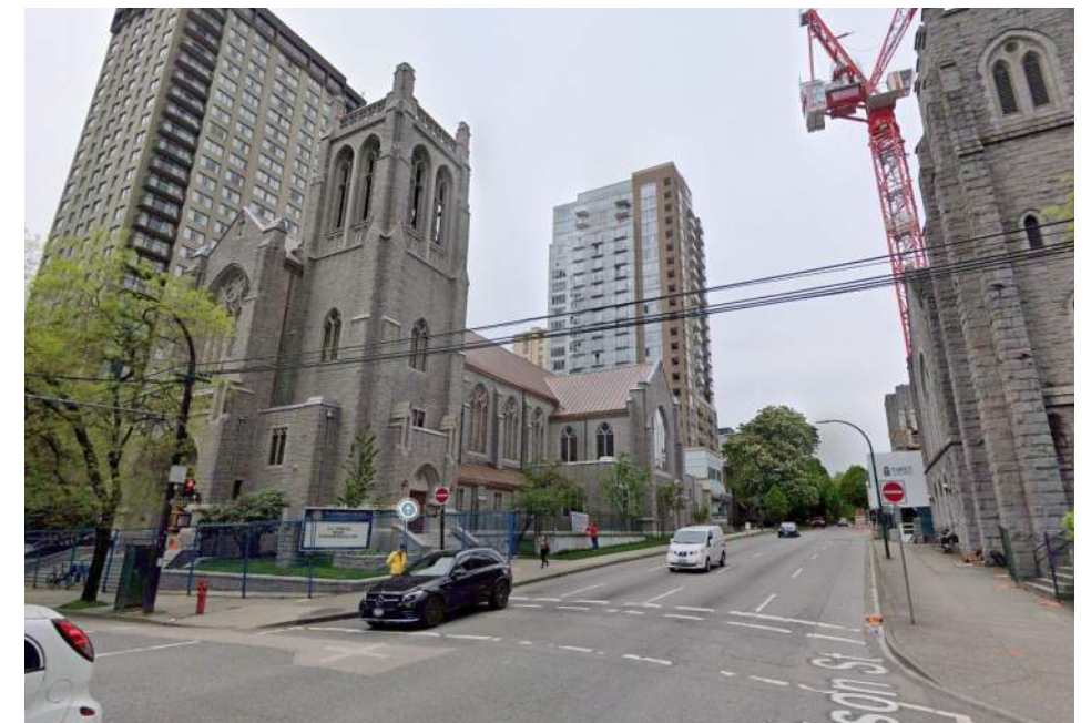
O. Burrard St and Nelson St frontages of St. Andrew's Wesley United Church at 1012 Nelson St. Church is to be integrated into the future development of The Butterfly Development .
