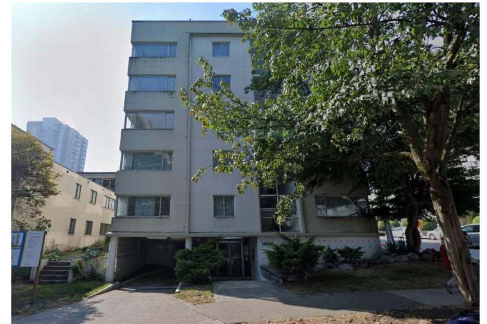
L. Barclay St frontage of a 6-storey residential building.
