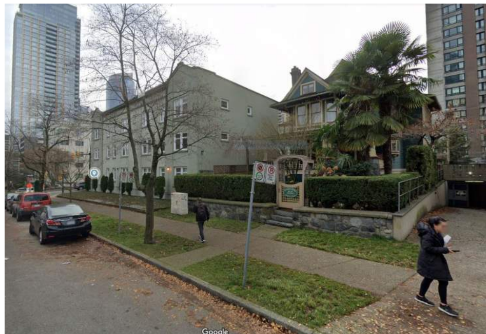
M. North elevation of O Canada House (right), a Bed and Breakfast & Heritage building, and The Biltmore (left) at 955 Thurlow St.
