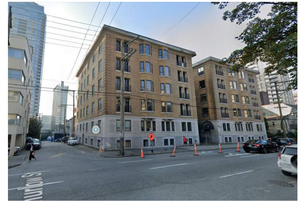
B. North elevation of Washington Court , a multi-family residential building at 998 Thurlow St.
