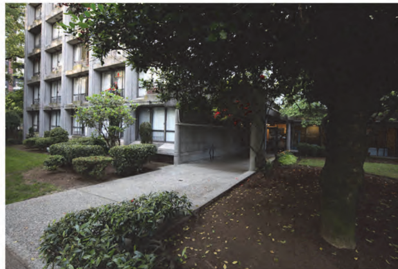
1031 Burnaby St - Residential Entry and Facade
