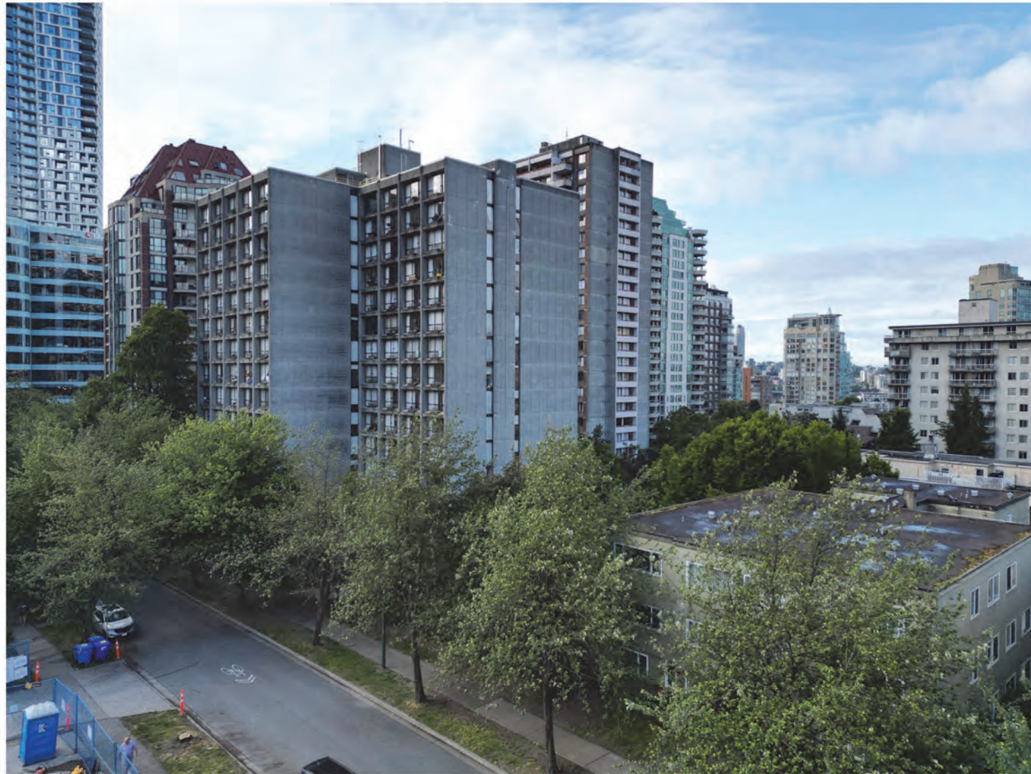
1031 Burnaby St - Overhead View
