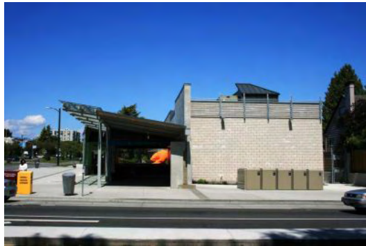
Langara 49th Canada Line Station
